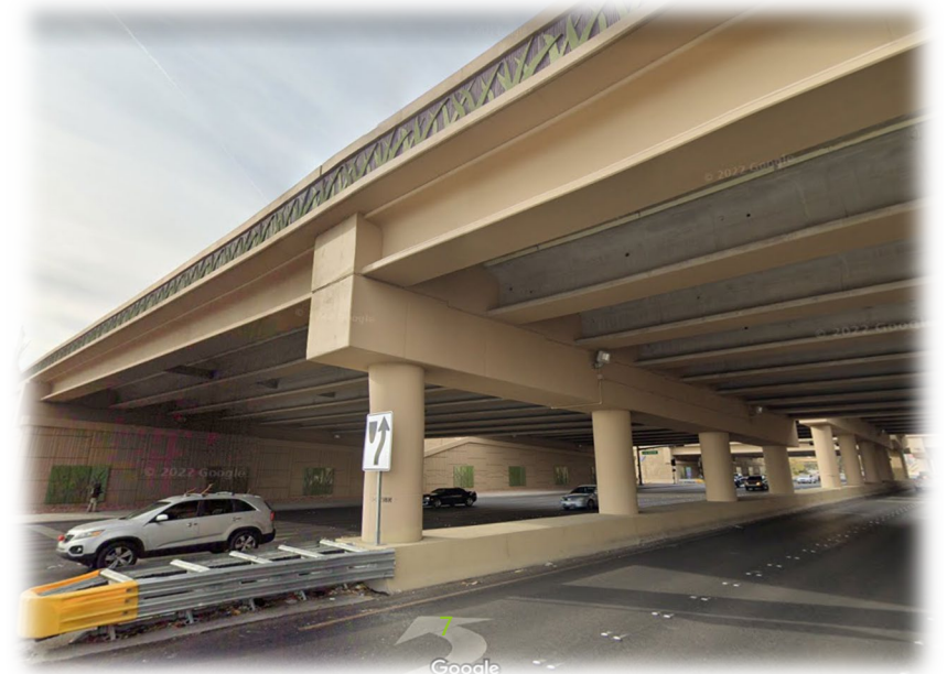
Precast Girders - Project NEON (Las Vegas) No Columns for Arlington Bridges
