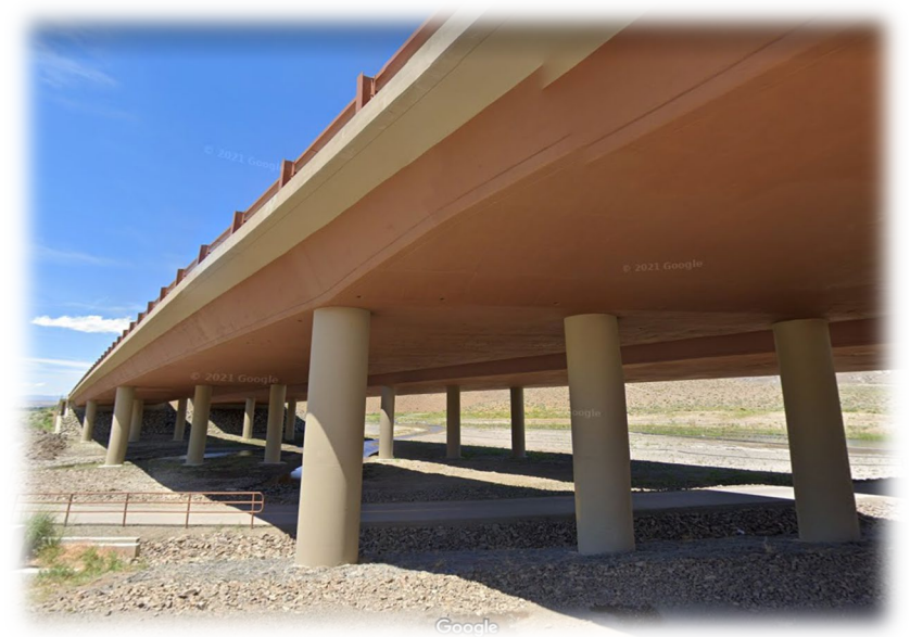
CIP - Box Girder From Veteran's Parkway (Reno) No Columns for Arlington Bridges
