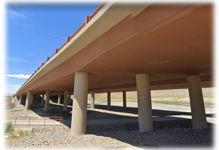
CIP - Box Girder From Veteran's Parkway (Reno)
