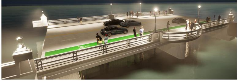
End Pylon Option 4 with Custom Luminaires and Forms+Surfaces LED Post-Top Luminaire on Mid-Bridge Pilasters and Under Top Rail Lighting ARLINGTON A V E N U E BRIDGES PROJECT
