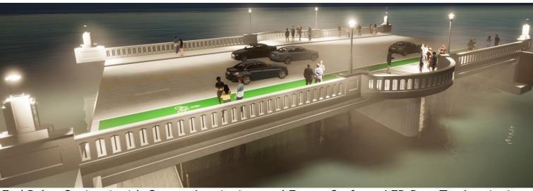
End Pylon Option 1 with Custom Luminaires and Forms+Surfaces LED Post-Top Luminaire on Mid-Bridge Pilasters
