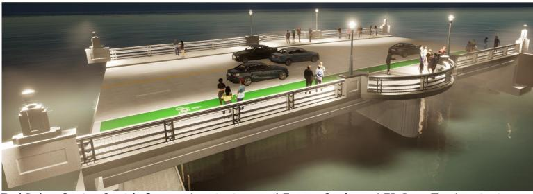
End Pylon Option 3 with Custom Luminaires and Forms+Surfaces LED Post-Top Luminaire on Mid-Bridge Pilasters and Under Top Rail Lighting
