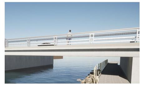
Option 2A - Metal Vehicular Bridge Rail with Metal Pedestrian Fence - Chevrons Up
