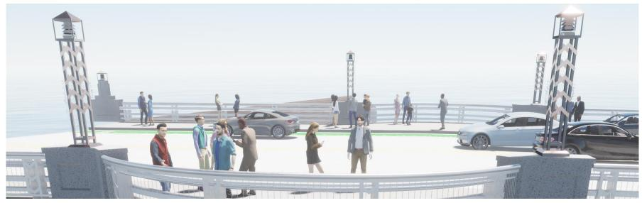
Option 2 - Custom Riverwalk-Inspired Column Mounted Luminaire with 14' Mounting Height on Mid-Bridge Pilasters
