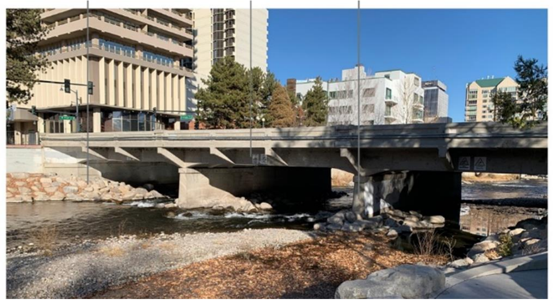
Existing North Bridge
