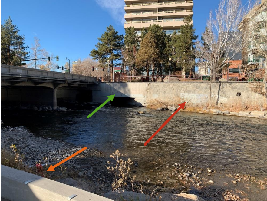
North Bridge - Existing
