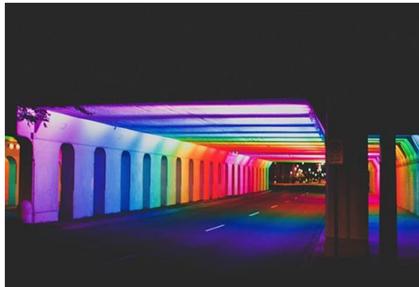
UNDER BRIDGE RGBW LIGHTING
