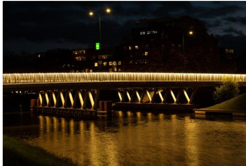
UNDER BRIDGE UPLIGHTING
