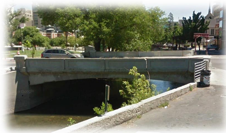
Existing South Bridge
