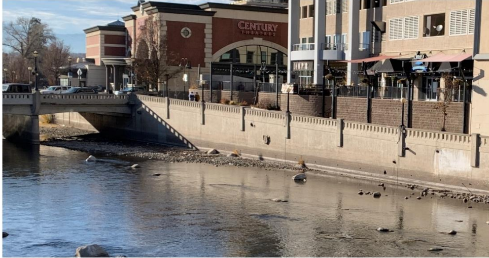
Repeat Existing Flood Wall Texture North Side
