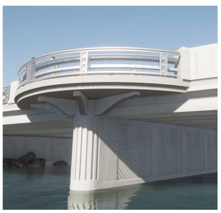
Option 2 - Overlook with Metal Vehicular Bridge Rail/Pedestrian Fence/Overlook, Concrete Brackets and Center Pier Treatment (layered)
