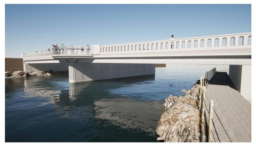
Overall Bridge Option 3 - Concrete Vehicular Bridge Rail with Metal Overlook Fence, Layered Motif
