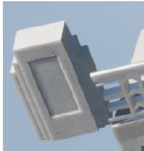
Group A: Tall End Pylon (3'-4" W x 2'-0"D x 5.0' H)
