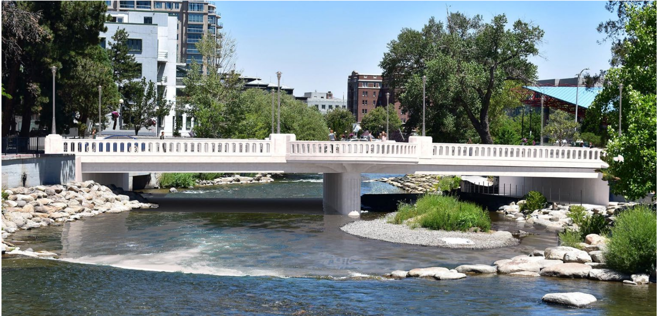
Option 1 - Texas DOT Concrete Bridge Railing
