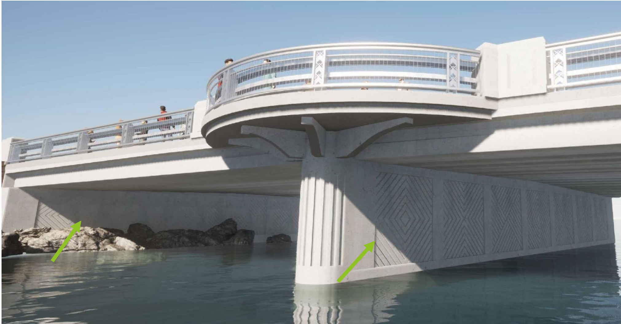
Pier and Abutment Wall Texture Coordinated with Railing Motif
