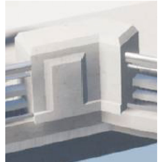
Group B: Short End Pylon (3'-8" W x 2'-6"D x 4'-6"H)
