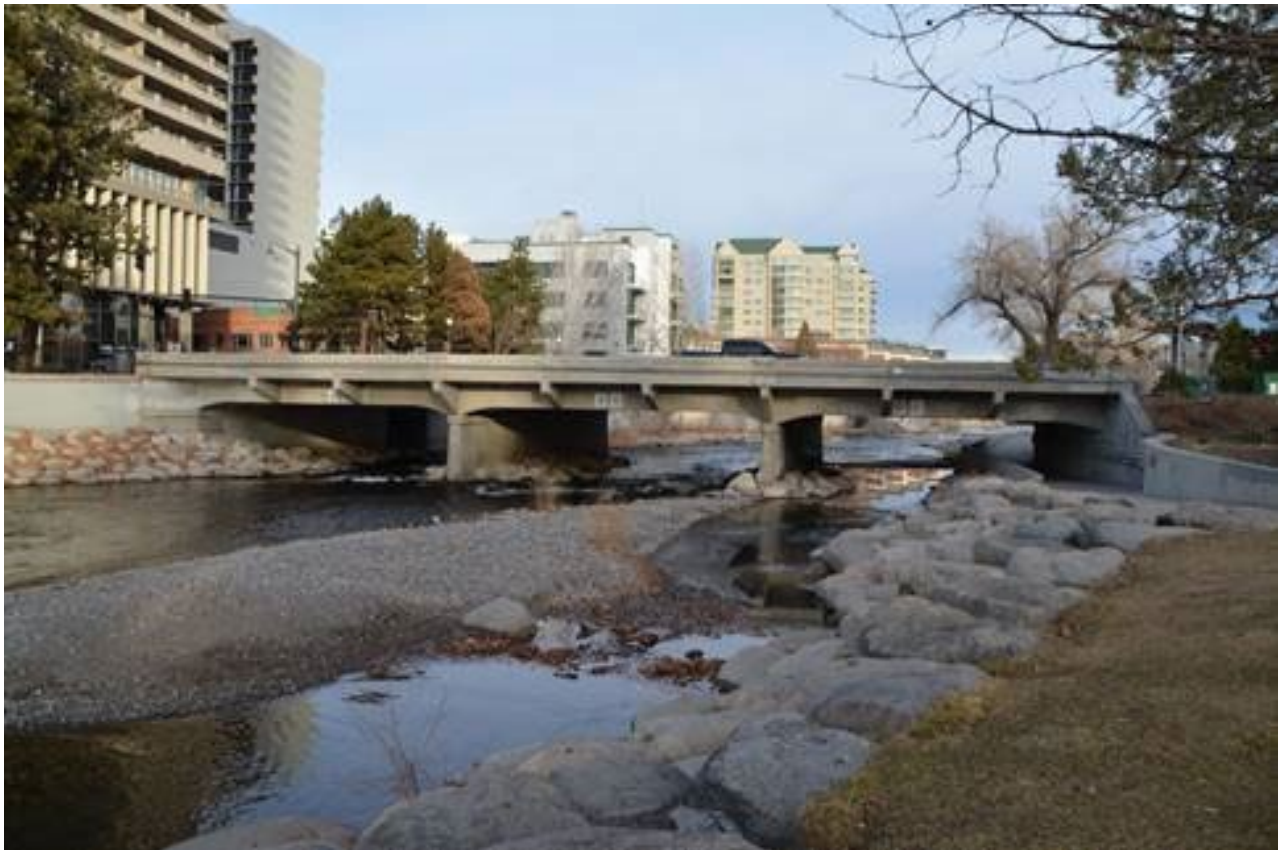
Existing Three Span (Two Pier) North Bridge
