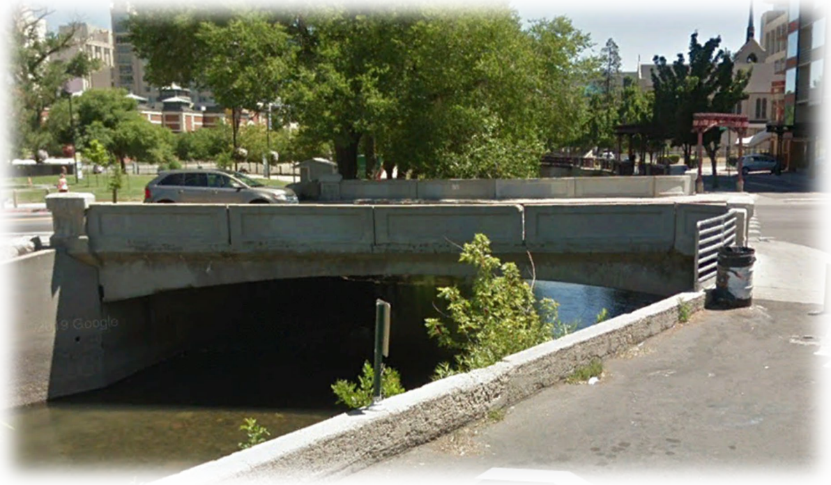
Figure 3. Existing South Bridge
