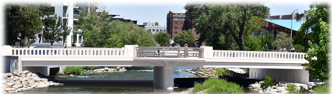
Figure 6. Hybrid Concrete with Metal Railing at Overlook
