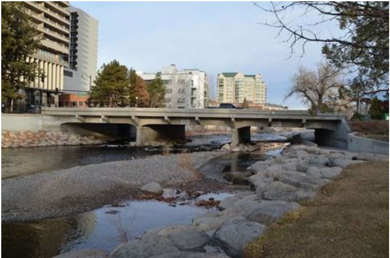
Existing Three Span (Two Pier) North Bridge
