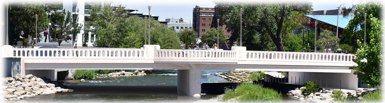
Figure 4. Texas DOT Concrete Railing
