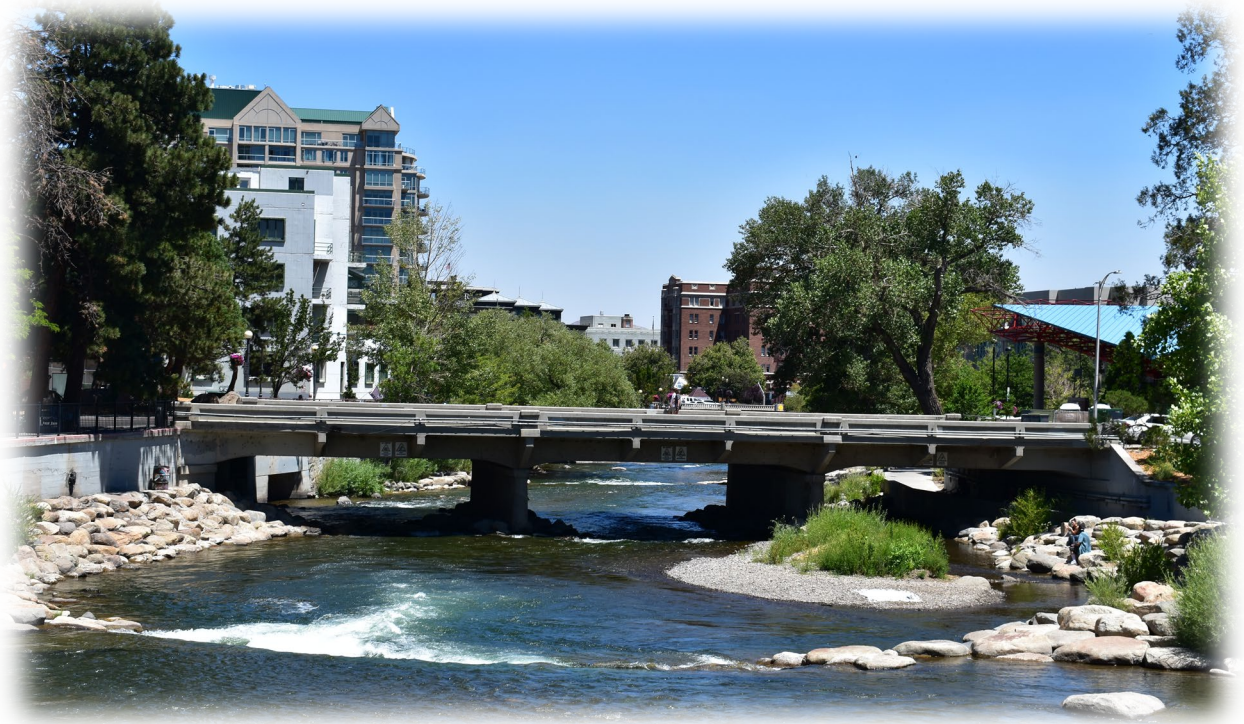
Figure 2. Existing North Bridge
