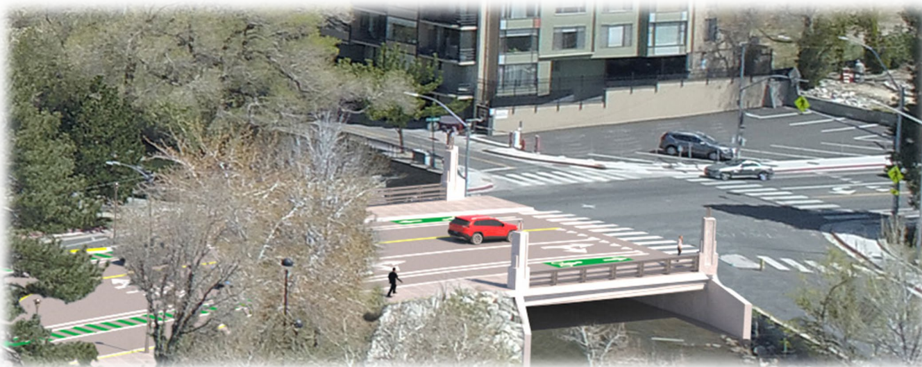
Figure 14. South Bridge Blow-up
