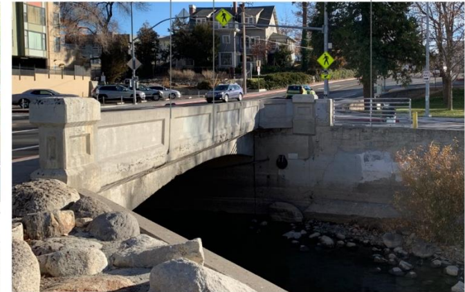
VIEW OF SOUTHERN BRIDGE
