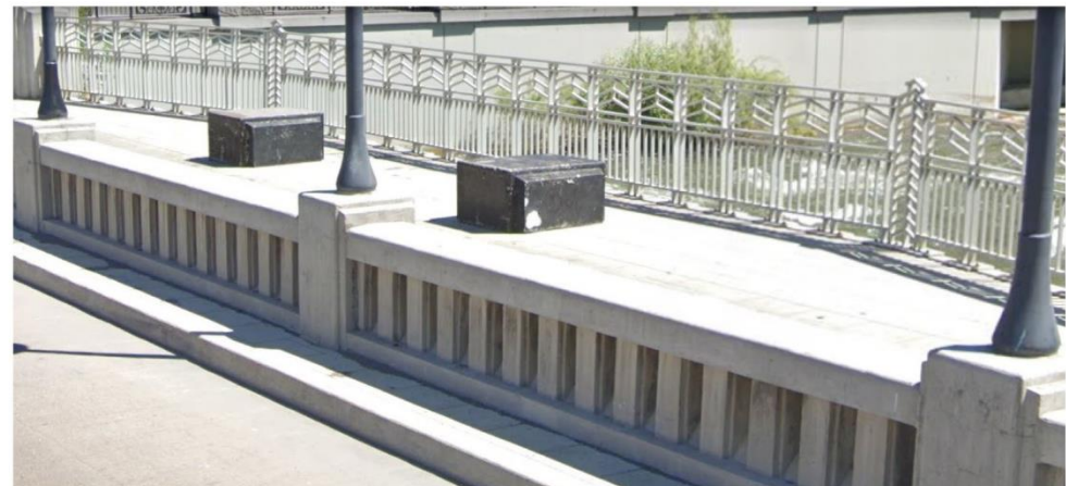
DECORATIVE RAILING AND GUARDRAIL
