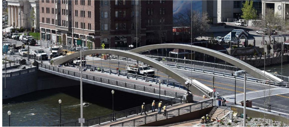
VIEW OF BRIDGE
