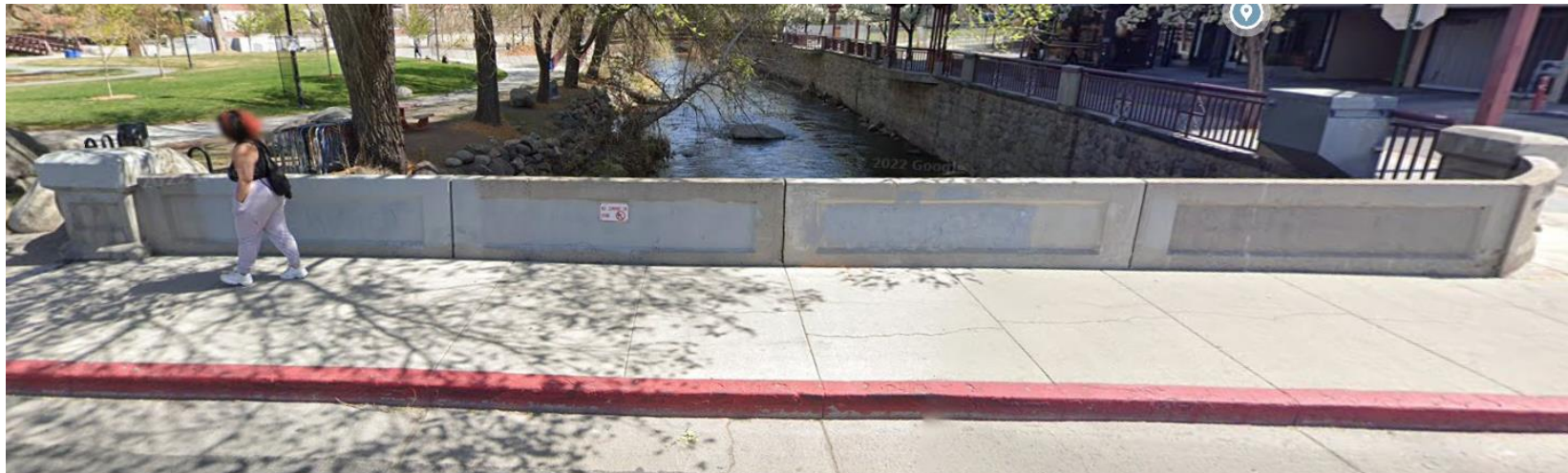
Arlington Avenue - South Bridge Concrete Parapet
