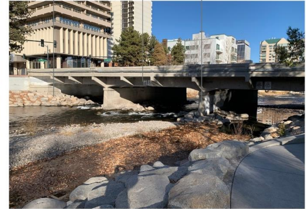
VIEW OF NORTHERN BRIDGE
