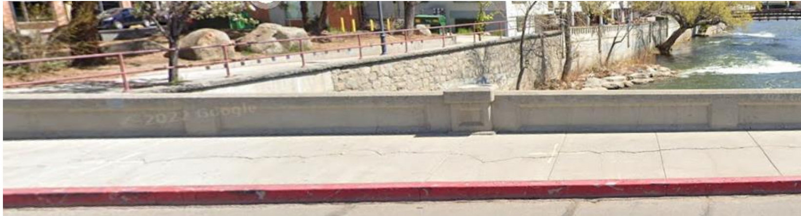
Arlington Avenue - North Bridge Concrete Parapet
