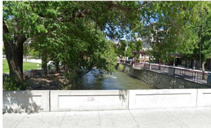
SOUTHERN BRIDGE SECTION, LOOKING EAST
