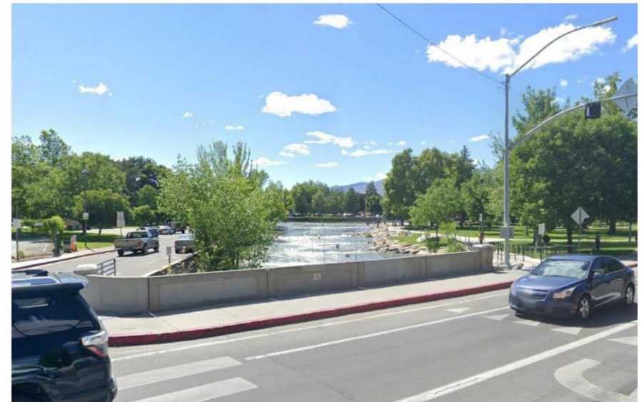
SOUTHERN BRIDGE SECTION, LOOKING WEST
