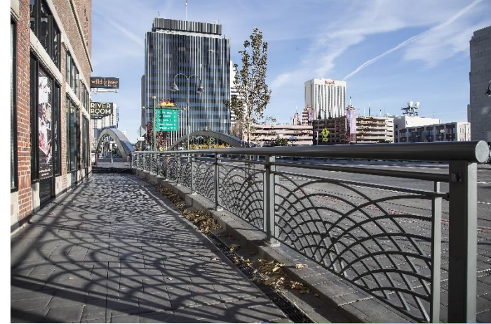
Off Bridge Pedestrian Fence and Rail
